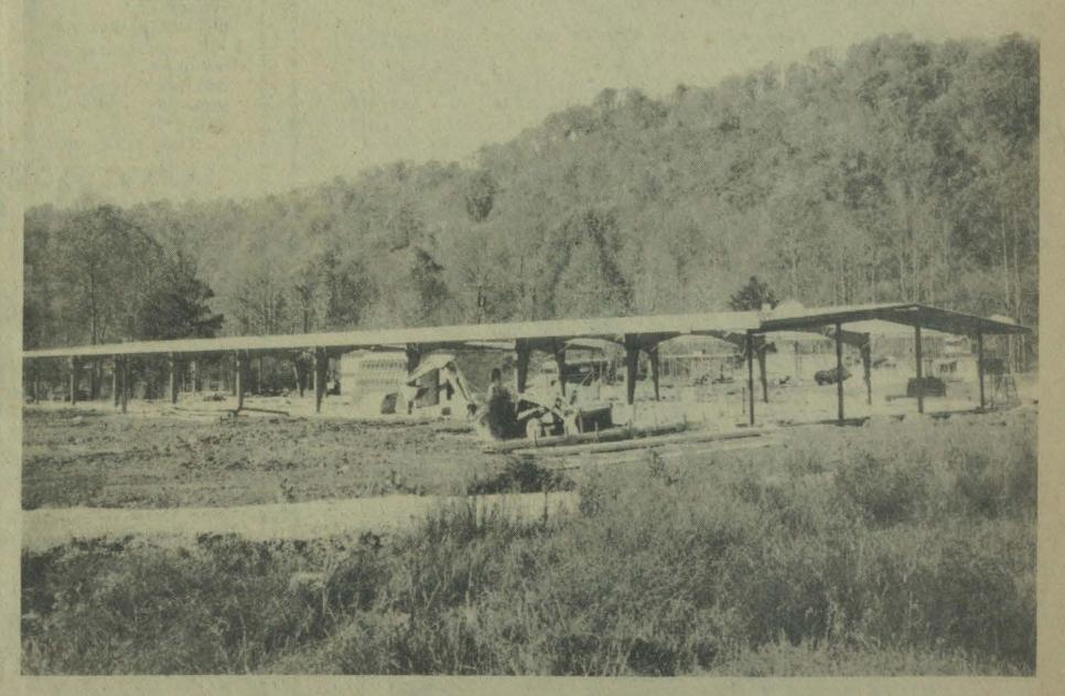
Steel is going up on the Island Creek Coal Company office building, near Combs Airport. The steel and brick structure will house an office force of about 75 persons and will be the center for direction of company coal operations in the area. A helicopter pad will be located at the rear of the building, it was said.
