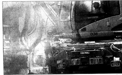
A typical drilling operation makes necessitates closing the road to all traffic. The drilling rig itself takes up almost two lanes. It takes about 10 minutes to drill one hole and place a length of railroad steel inside.
