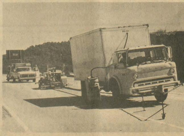
REFLECTOR STUDS being installed on new U.S. 23, near Allen. The studs, which have been placed on most of the county's larger roads, are designed to help orient motorists, especially on dark, rainy nights.
